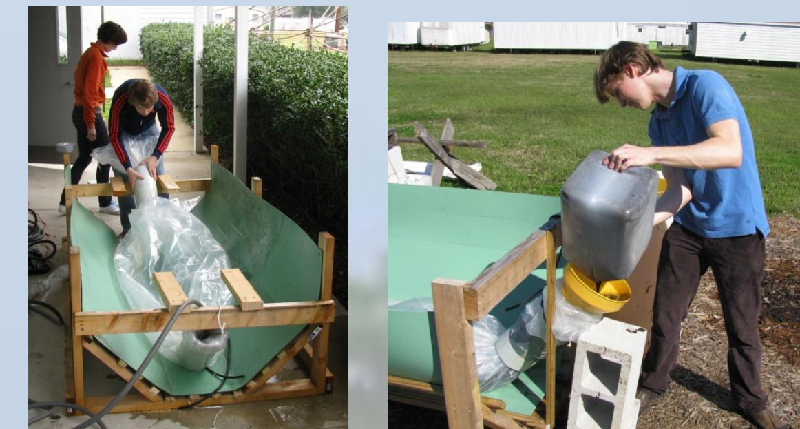
Construction of and filling the bag anaerobic digester with pig manure slurry. Featured: Kelly Jones, past project lead, and Rachel Donahue, previous team member
